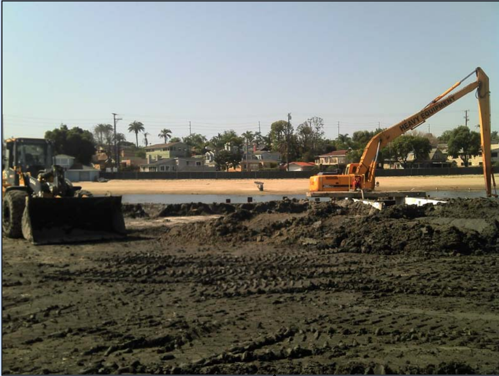
Photo on previous page: the AIS dredge on the water at the Lagoon with FOCL's East Bank Restoration in the background; Photo above: the staging area for the dredged sediment before it is taken to the Port of Long Beach; Photo below: an automobile engine pulled up from depths of the Lagoon. All photos from Dave Pirazzi.
